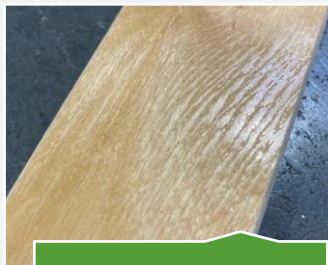
rough surface up to 10% of the surface, up to 0.3mm in depth
